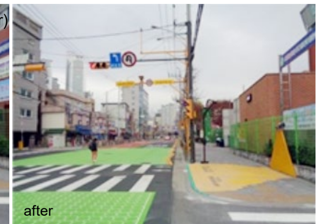
Applying anti-slip facilities (before & after)
